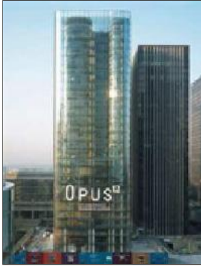
Opus 12 tower, La Defense, Paris, France. Architects: Valodé & Pistre
